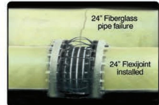
The expansion or contraction of a rigid pipe section that is restrained at both ends will generate a force equal to that required to compress the pipe from its expanded length back to its original length. These forces can be very high and can cause the piping to buckle, compressive failure of the piping or even damage to other equipment.
